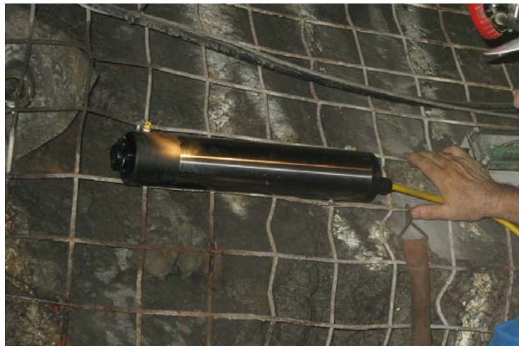
TOP Logger shackled to wire mesh using eye bolts
